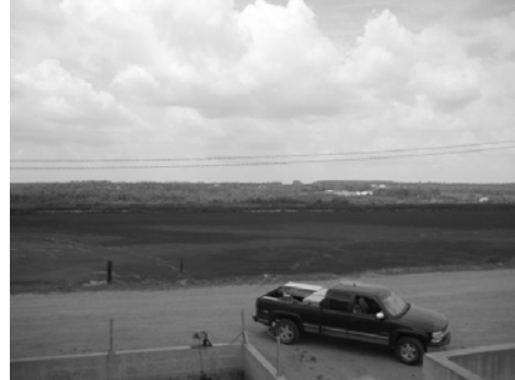
The System – Collection Pit
