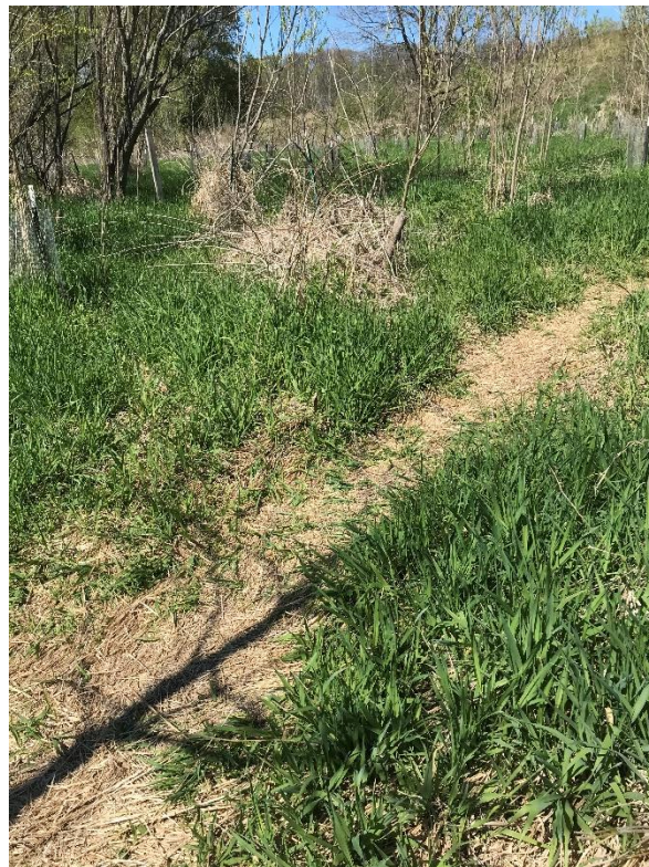
Image 6. Straw provides a barrier to soil in FP7.
